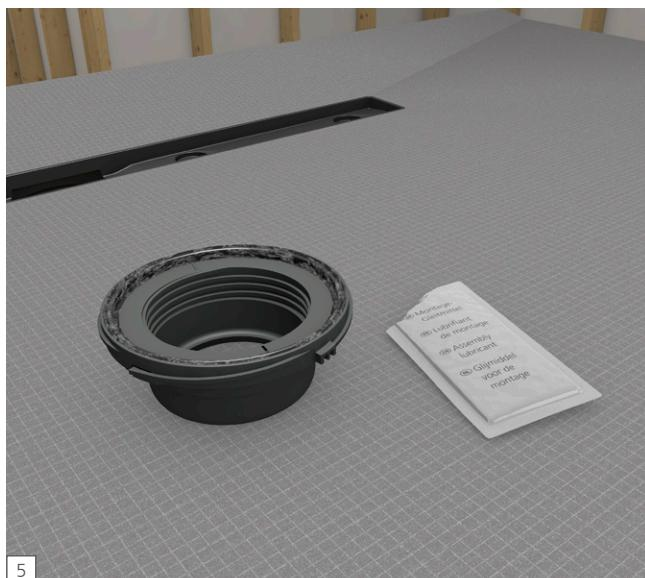
**EN** Apply the wedi provided safe lubricant to the black rubber ring inside the wedi Drain Body.
